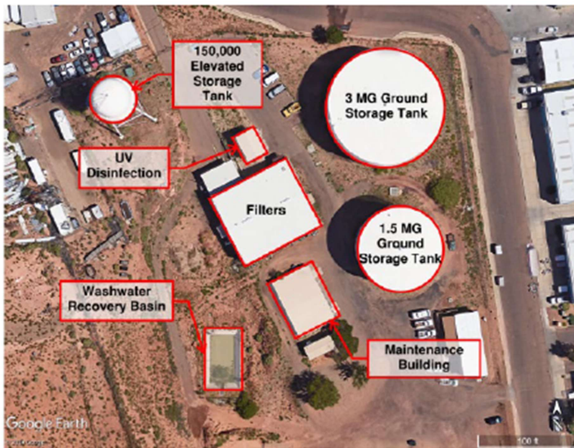
Figure 1 Current WTP Aerial Photo
